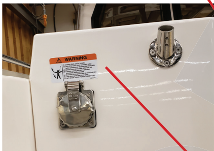
Shock & Fire Hazard
